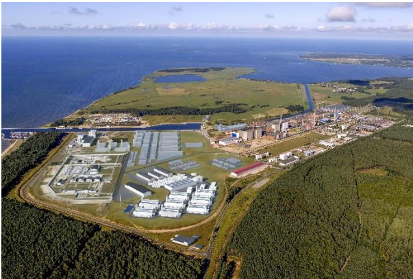
Aerial view with visualisation of the hydrogen hub in Lubmin with planned large-scale PtX Development electrolyser plant. © PtX Development
